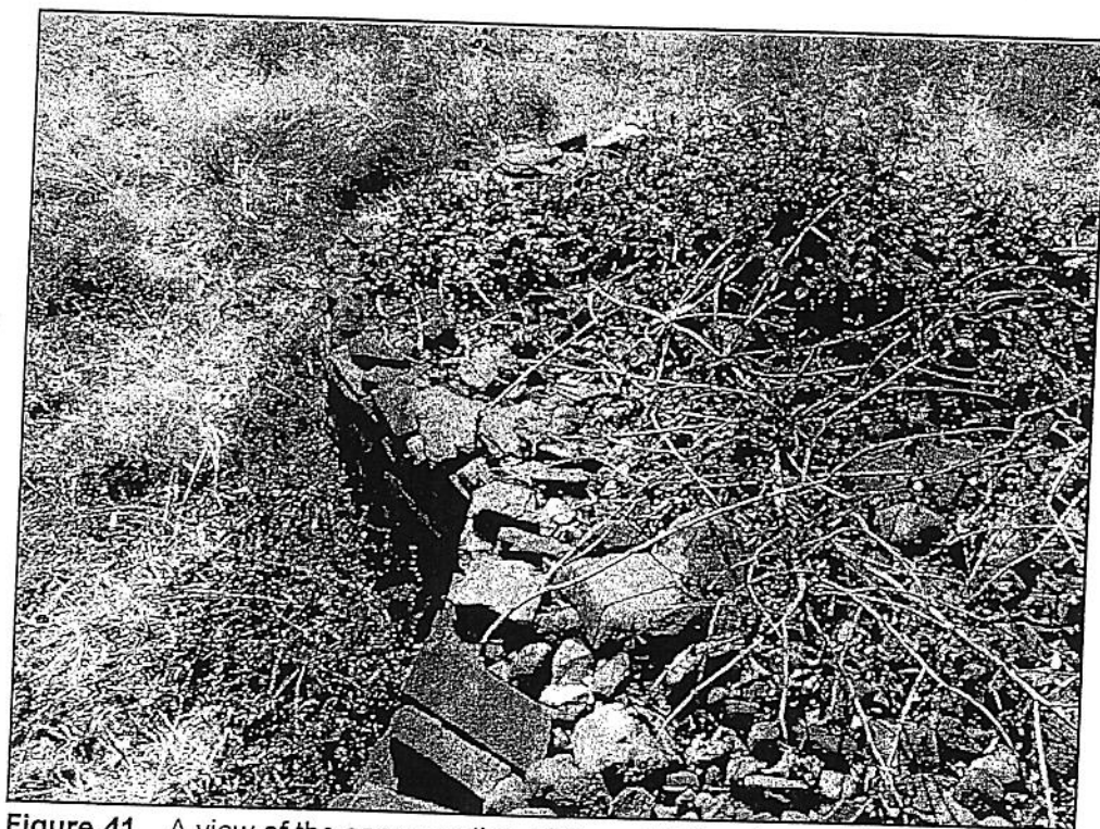
Figure 41 A view of the same section of the wall taken from above. The junction and artificial rounding can be clearly seen. The reconstruction would follow the outline of the original foundation. A herbicide would also need to be applied to eradicate any vegetation growing in the walls. See figure for information about reconstruction.
