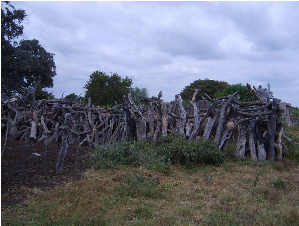
The erection of this kraal at Norma A was informed by the Indigenous Knowledge System (IKS). Note the closeness of the logs, dug into the ground without anything tying them together.
