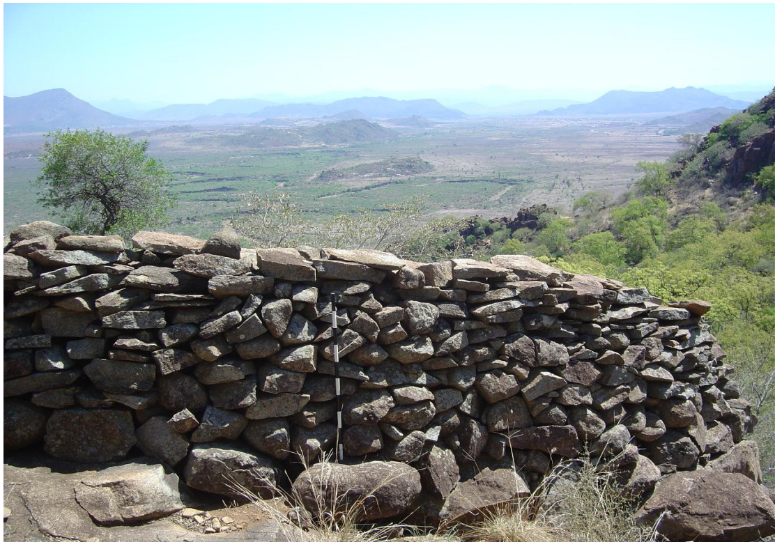
2. Well preserved wall on northern side of Mosego
