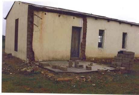
Figure 2 Visible wall marks and the slab foundation of the dilapidated covering.
