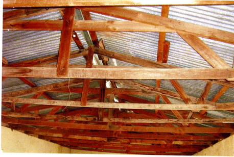
Figure 5 The rafters and corrugated iron form part of the roof refurbished in 1952
